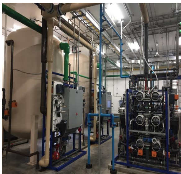
Figure 3: Delco Water biofilters and reverse osmosis/nanofiltration skid at Montana First Nation
